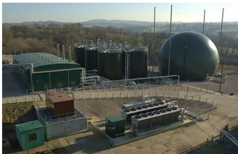
Figure 2 – The built Blackburn Enhanced Enzymic Hydrolysis project
